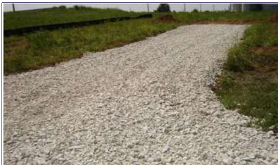
Figure 8.1: Temporary access track
